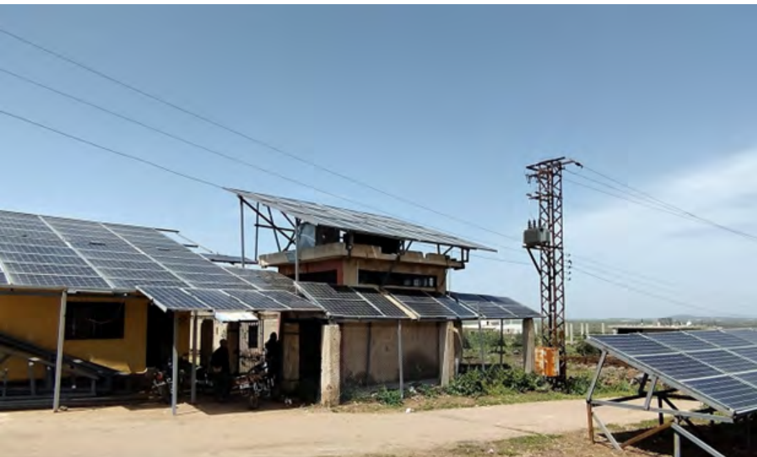
Solar system on a rehabilitated water well in Hara township, Dar'a. (Source: CA-SYR)
