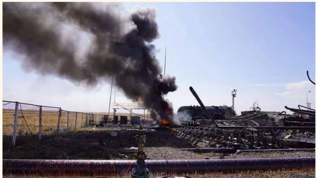
As-Sweidiyeh gas-powered electricity station (Source: North Press Agency )
